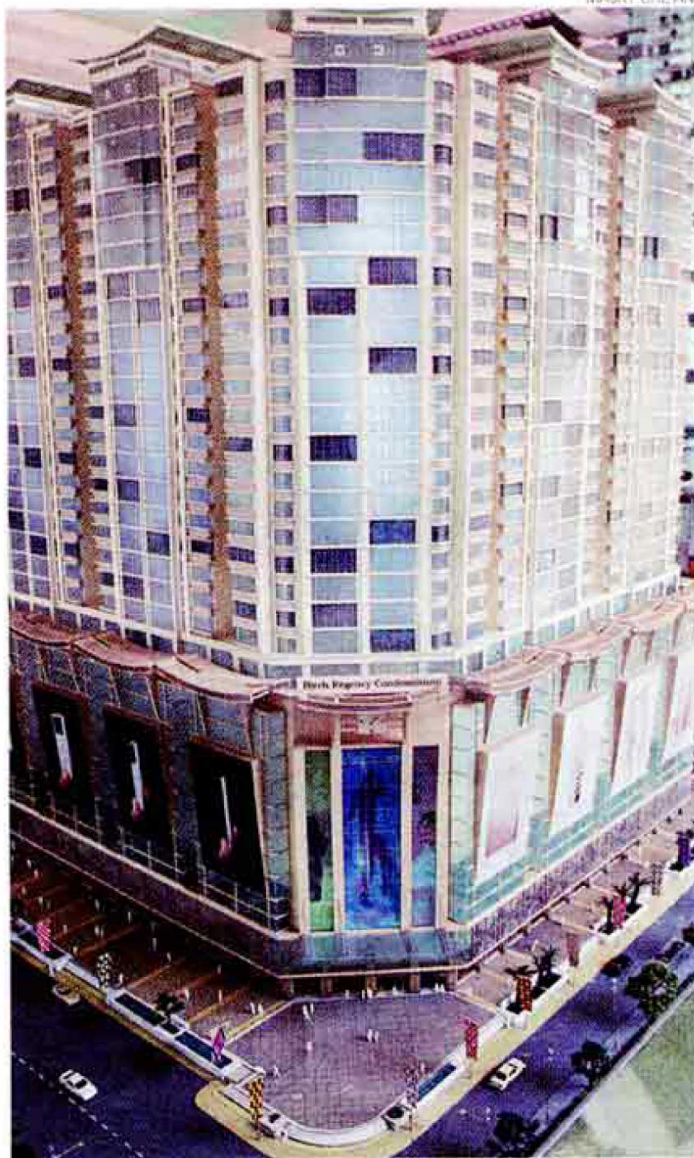
Work on the RM1-billion project has already begun
